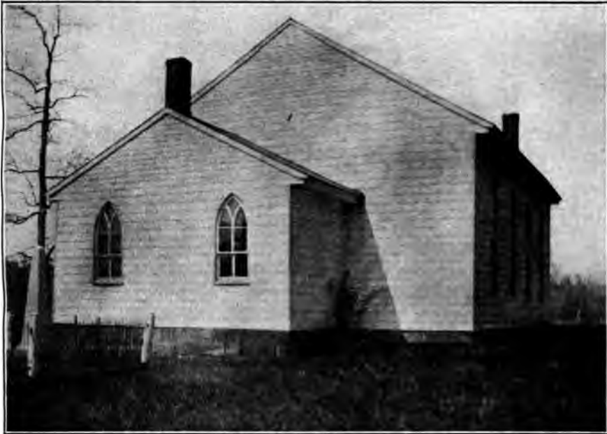
ST. JAMES'S CHURCH, CROSS CREEK, BUILT 1861.
